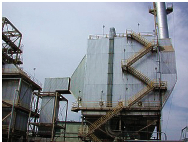
Figure 2-3.4: Electrostatic precipitators remove particles before they are released into the air.
